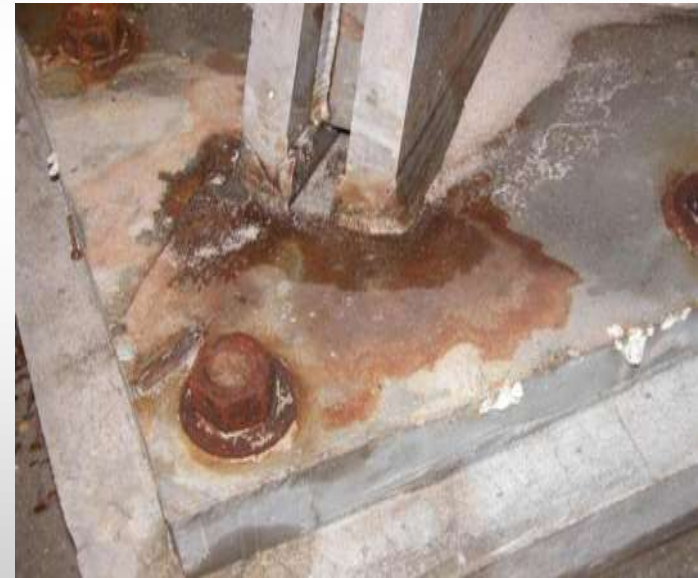
Stainless steel plate/galvanized steel fasteners
