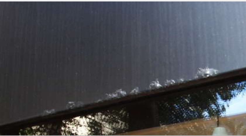
Peeling painted Aluminum Florida, <10 yrs
