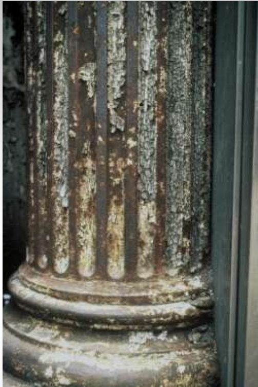
Peeling painted carbon steel
