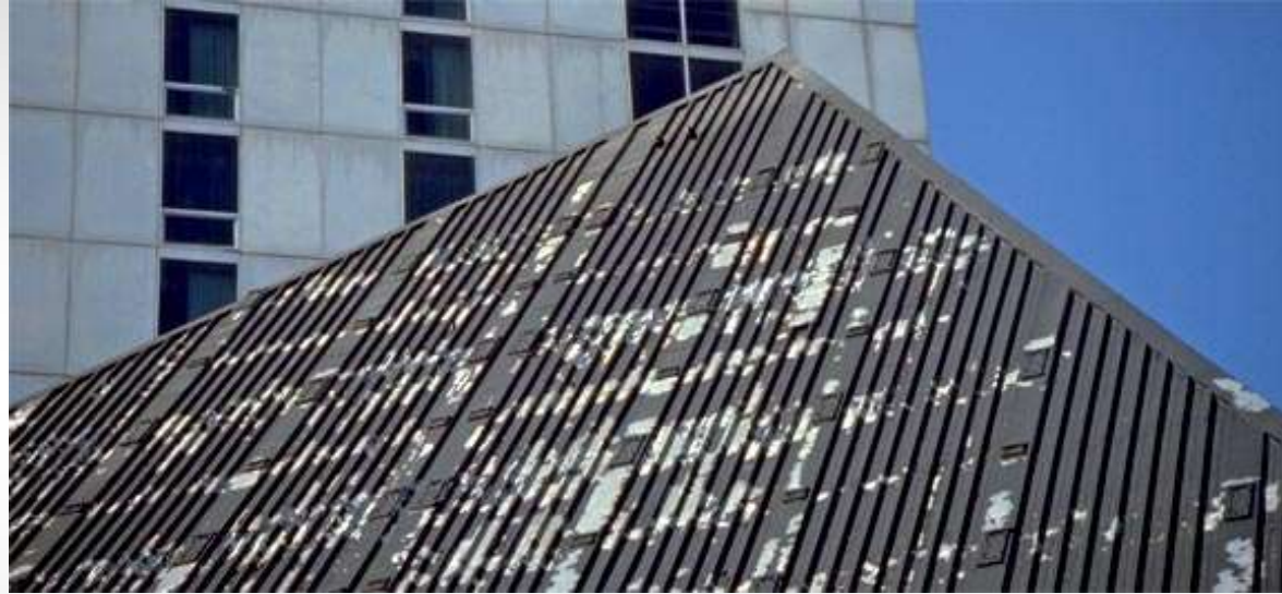
Peeling painted aluminum roof, 25 years
